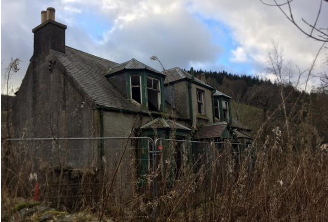
Figure 13: Image of the existing Dwelling House
