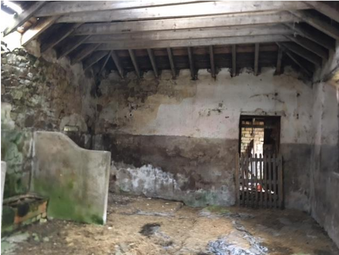
Figure 15: Existing Steading Interior
